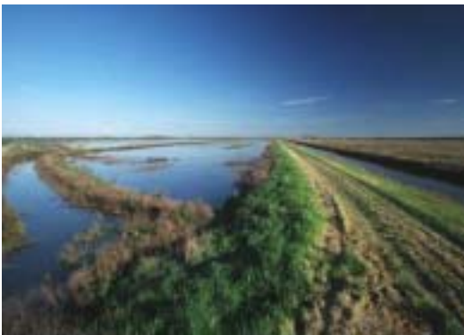
WETLANDS RESTORED FOR FLOOD MANAGEMENT
