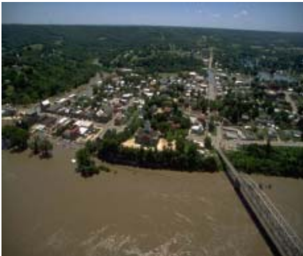
AERIAL PHOTO OF GREAT MISSISSIPPI FLOOD
