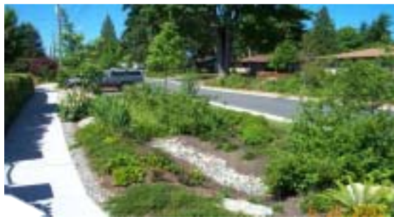
STREET SWALE IN SEATTLE
