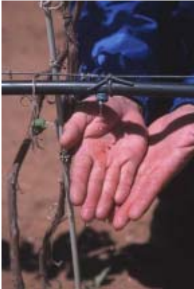
DRIP IRRIGATION SYSTEM
