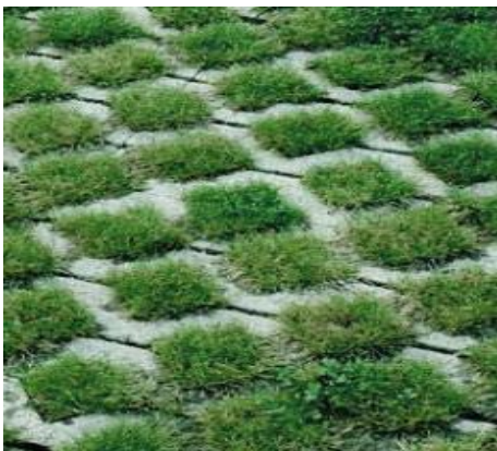
EXAMPLE OF PERMEABLE PAVEMENT
