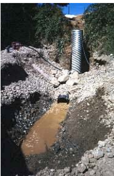
INFILTRATION GALLERY DURING CONSTRUCTION ON SUCKER CREEK, OR
