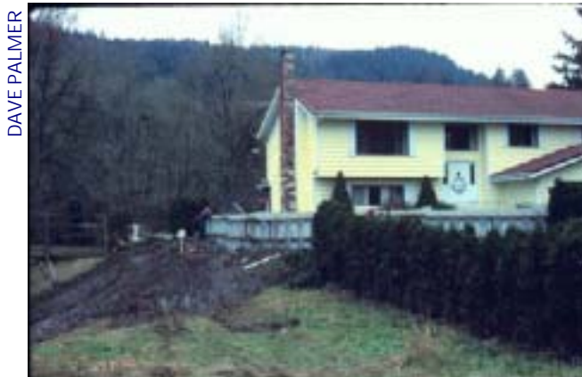
FLOOD WALL BEING ERECTED FOR PRIVATE LANDOWNER
