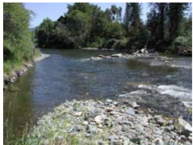
SITE OF A FORMER IRRIGATION PUSH-UP DAM REPLACED WITH AN ALTERNATIVE DIVERSION STRUCTURE
