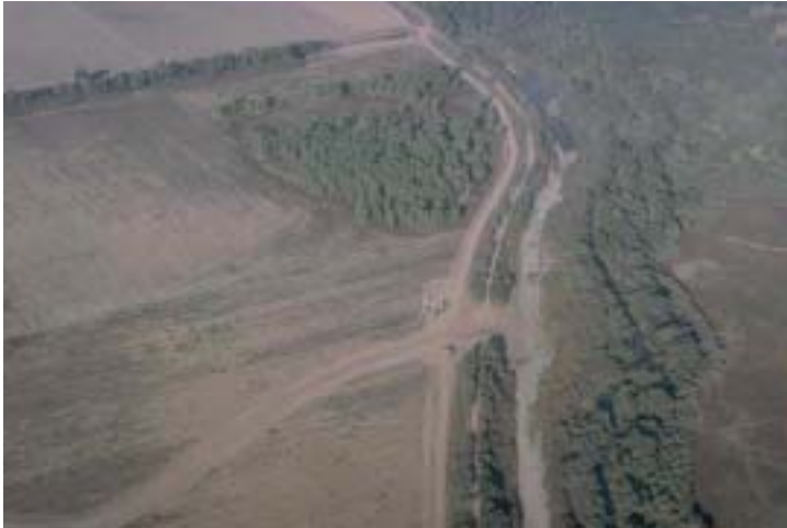
INITIAL BREACH ON THE CONSUMNES LEVEE IN OCTOBER 1995
