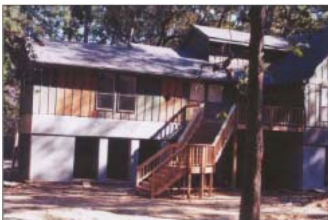
EXAMPLE OF FLOOD PROOFING THROUGH ELEVATION
