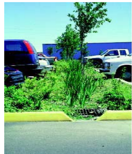
PARKING LOT SWALE FOR GROUNDWATER REPLENISHMENT AND CAPTURING RUNOFF
